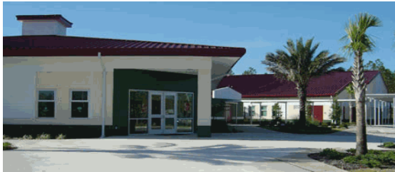
Timberlin Creek Elementary School 555 Pine Tree Lane St. Augustine, FL 32092
